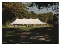
A traditional pole tent is erected using center poles to push up the canopy. The tent is then stabilized with guylines at each of the side poles. Because the guylines must be staked into the ground, this style tent requires an earthen or soft surface. We can install a pole tent on an asphalt surface and patch the stake holes upon removal of the tent. For a festive party atmosphere, a pole tent is the way to go.
