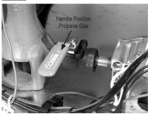
The handle must be fully set at 90 degrees to gas flow (propane gas) or parallel to gas flow (natural gas) for proper operation. Also refer to the decal located on the heater's base, adjacent to the selector valve.
